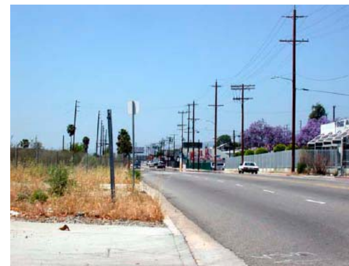
San Fernando Rd. at Parcel D looking N/W
